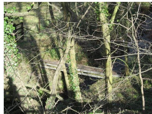
Image 07: Small bridge onto site across Crimple Beck
